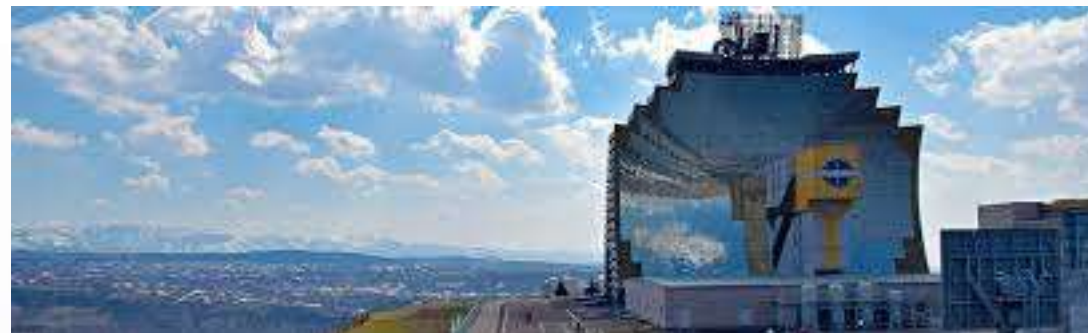
Institute of Solar Physics (Parkent) Unique scientific facility in solar energy and astrophysics
